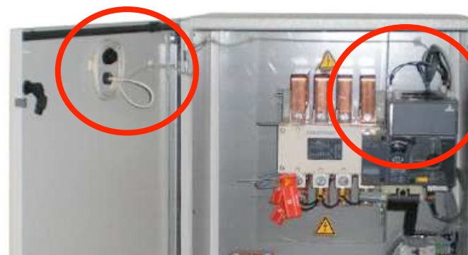
RJ45 PORT for ATyS D10 connection
